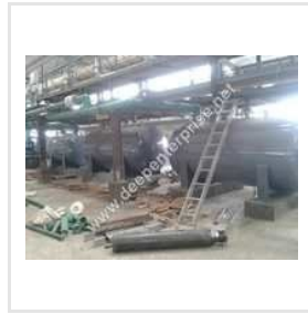
Resin Coating On M.s Tank
