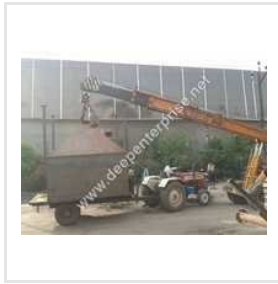
FRP Lining On MS Tank
